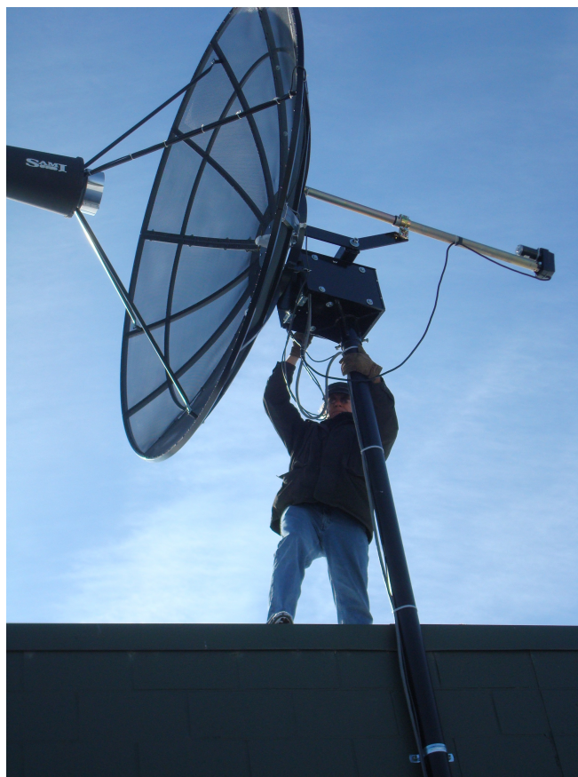
Illustration 1: FRCC SRT during installation and alignment.
